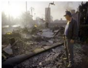
Damage caused by the 1994 Northridge earthquake.
